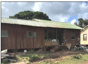
Kaipu Camp house #6 The first to undergo restoration
